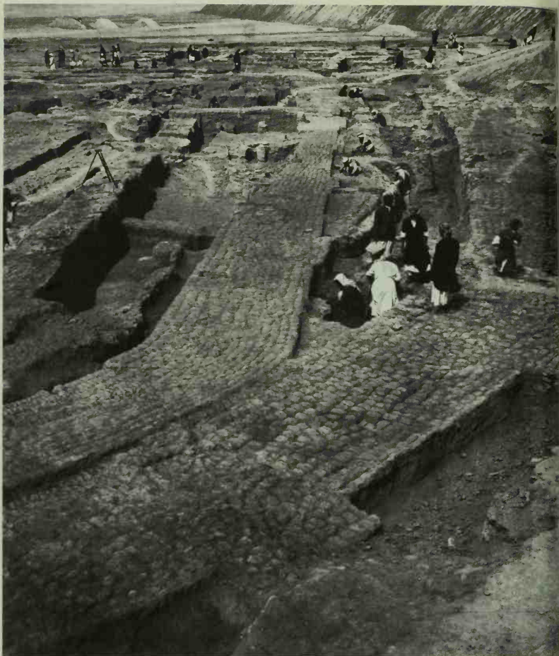
53 Excavating the foundations of the Oval Temple enclosure at Khafaje (looking northwest). The individual mud-bricks (of the 'plano-convex' type) had laboriously to be articulated. The excavators in the foreground have discovered the deposit of sand on which the foundations rested
