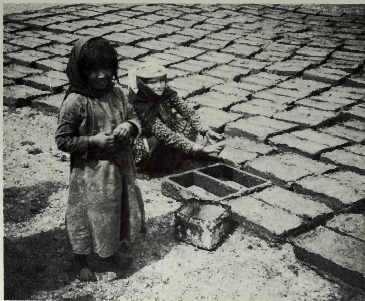
72 In the modern villages of Iraq bricks are made of mud, tempered with chaff and cast in a bottomless wooden mould, smoothed on top and dried in the sun
